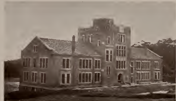
Underwood Hall, Rear Elevation
